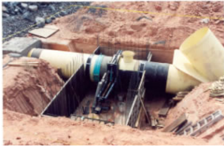
Fig 8. Construction of an outlet of horizontal drains
