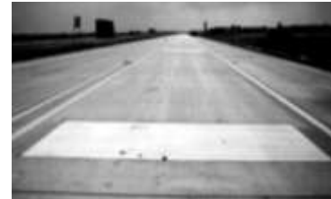
Figure 4 Transverse pavement marking in USA [19]
