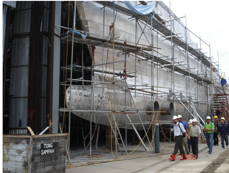
Figure 1.3 : Catamaran Boat Under Construction
