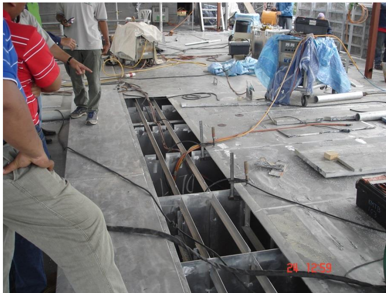
Figure 1.4 : Grillage Deck Structure
