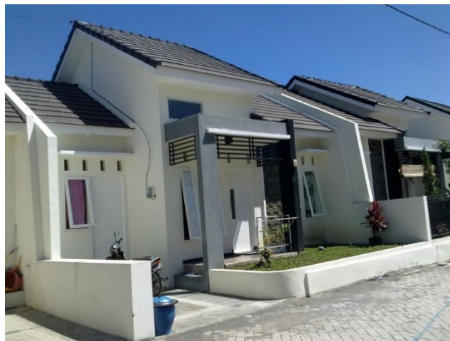
Figure 1 A single storey terraced house in Malang, used for field measurements
