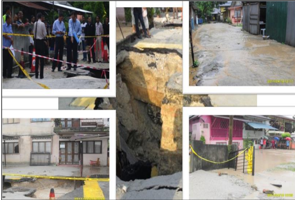
Figure 1.5: Sink Hole at Kg. Bharu
