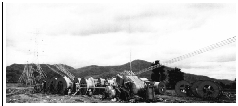
Figure 5. Conductoring a transmission line
