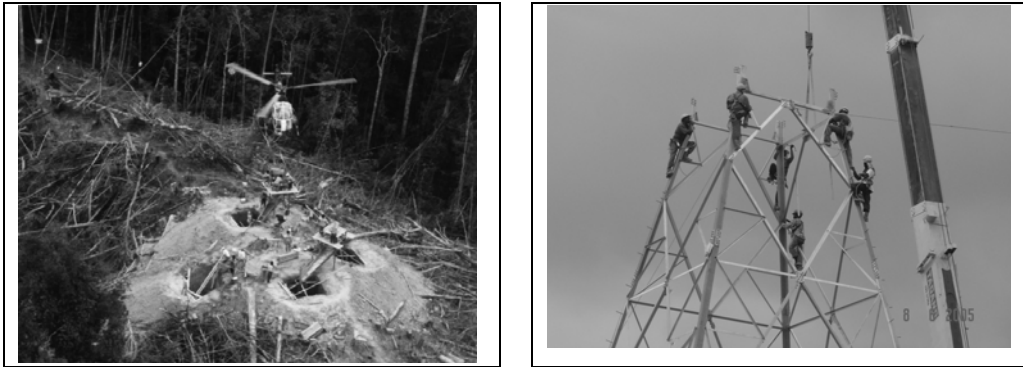
Figure 4. Foundation construction by helicopter (left), and tower erection by crane (right)
