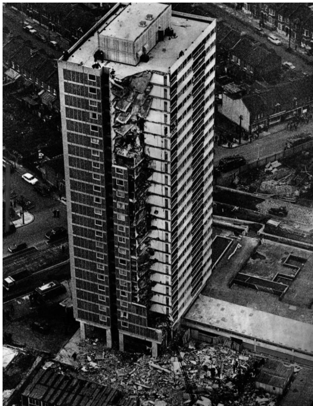
Figure 1.1 Partial collapse of Ronan Point apartment building
