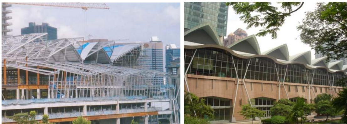
Figure 9 During and after construction of KLCC Convention Centre.
