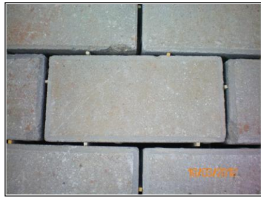
Figure 1 Bamboo sticks were used to uniform the joint width
