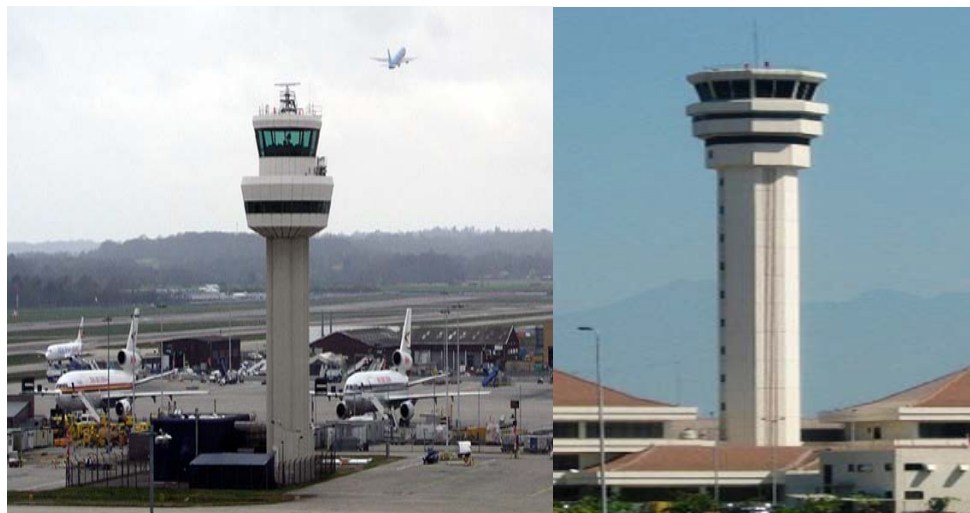
Figure 1.1 ATC tower's samples (Aviation, 2014)
