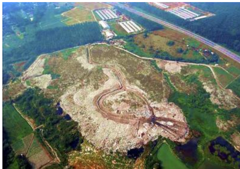
Figure 1.1 Cypark's solar plant under construction, next to the Pajam landfill
