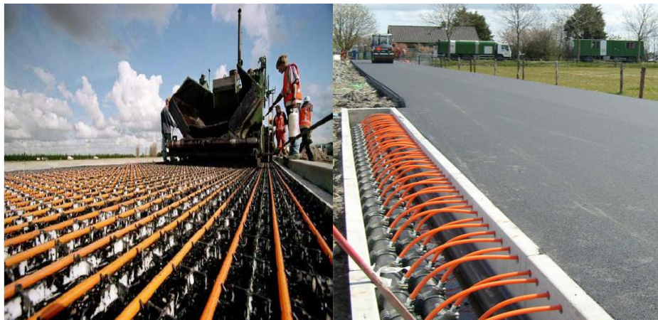
Figure 1.4 Roadway power systems
