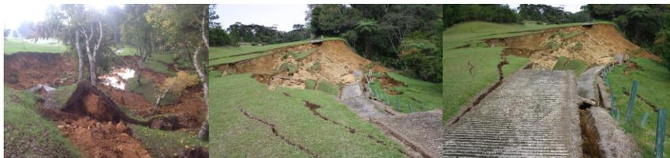
**Figure 1.** Ground failure after earthquake at Ranau, Sabah
