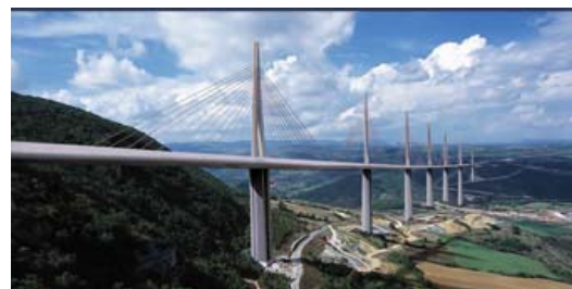
Figure 11: The Millau Viaduct at the Gorge du Tarn, France , 2004, by Norman Foster
