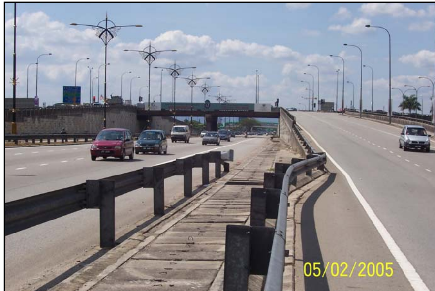
(a) Longitudinal View of the Bridge
