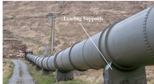
Fig. 1. Pipeline installed on the ground
