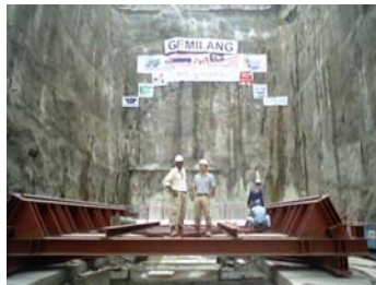
Figure 9: TBM Cradle
