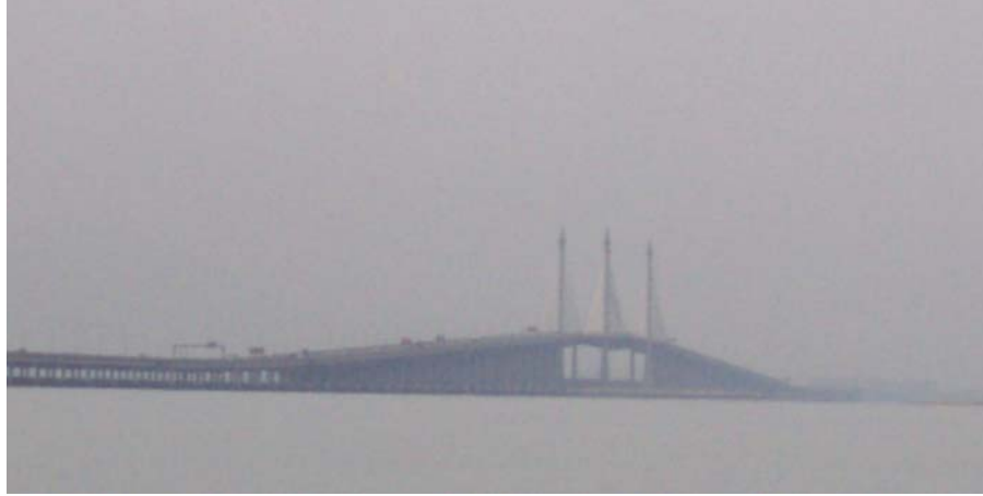
Figure 1: The Penang Bridge.
