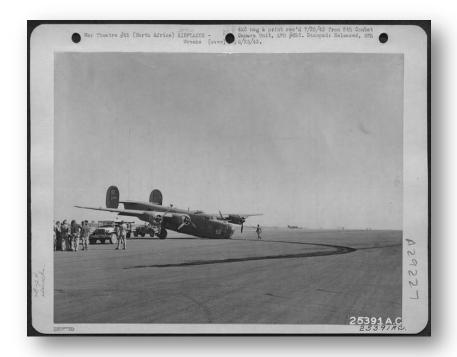
Fig 1.2: A B-24 Liberator, shown after suffering a nose wheel failure at a base in North Africa. Nose wheel shimmy was a serious enough problem that all the Halpro aircraft carried a spare nose wheel when they left Florida.
