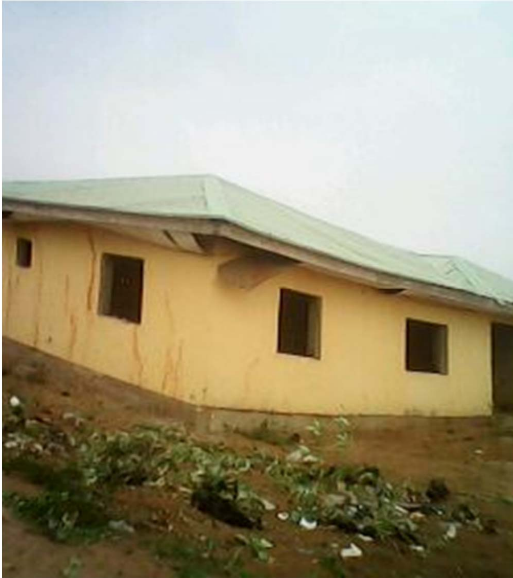
Figure 1.8: Scattered Refuse due Lack of collection and disposal point
