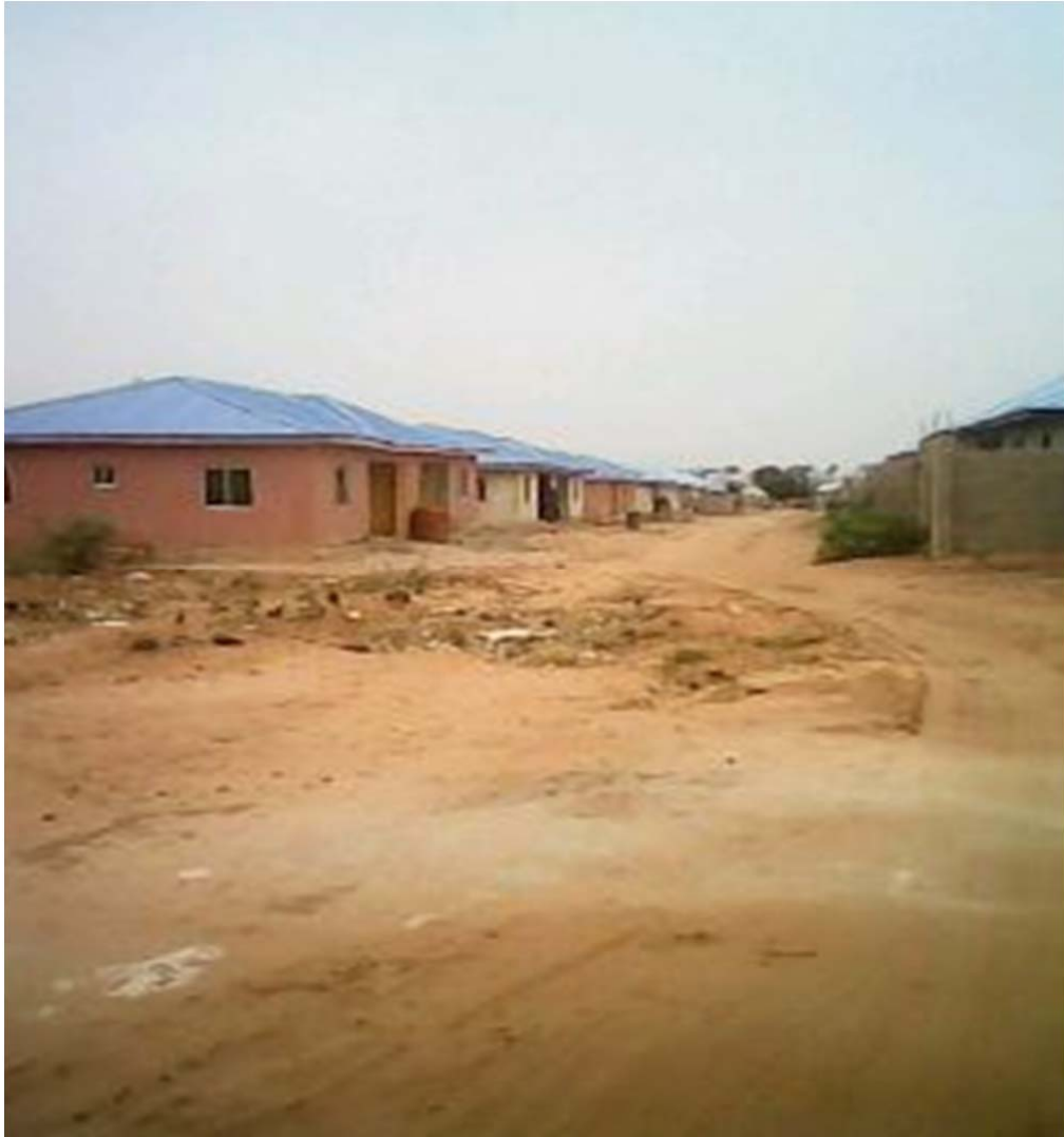
Figure 1.7: Poor Asses and Unpaved Road
