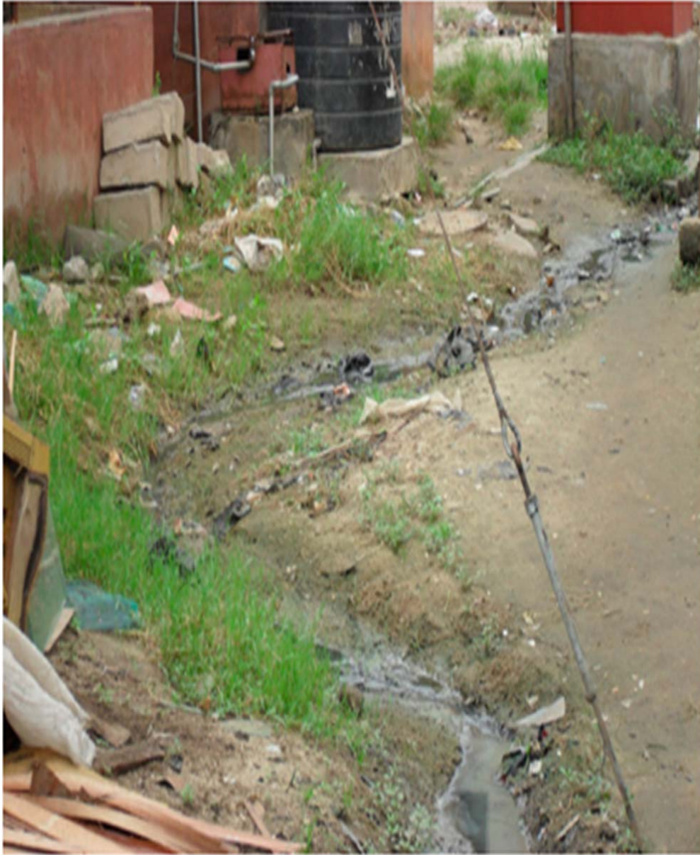
Figure 1.6: Exposed drains due to inadequate provision of drainage system
