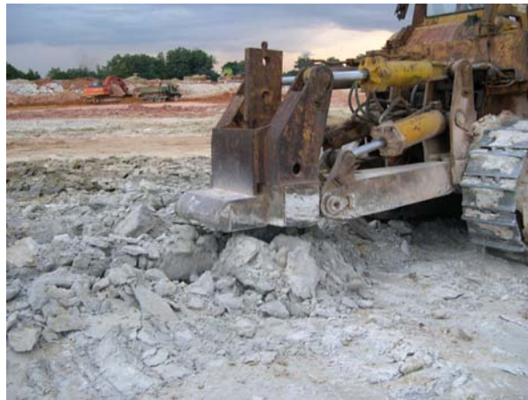
Figure 7.1: Ripping process at Line 1, Kempas
