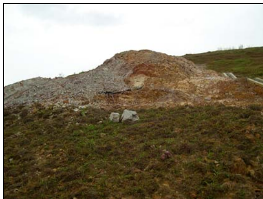
Figure 2.4 : Protruded rock mass at a slope that could not be ripped due to topographical factor (Location: Bukit Indah)
