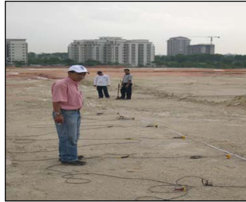
Figure 4.5 : Inspecting the seismic line before performing the test (Location: Desa Tebrau)
