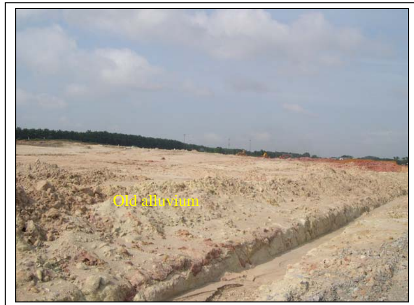
Figure 5.6 : Presence of old alluvium (whitish grey) in proposed site of Taman Kempas Indah
