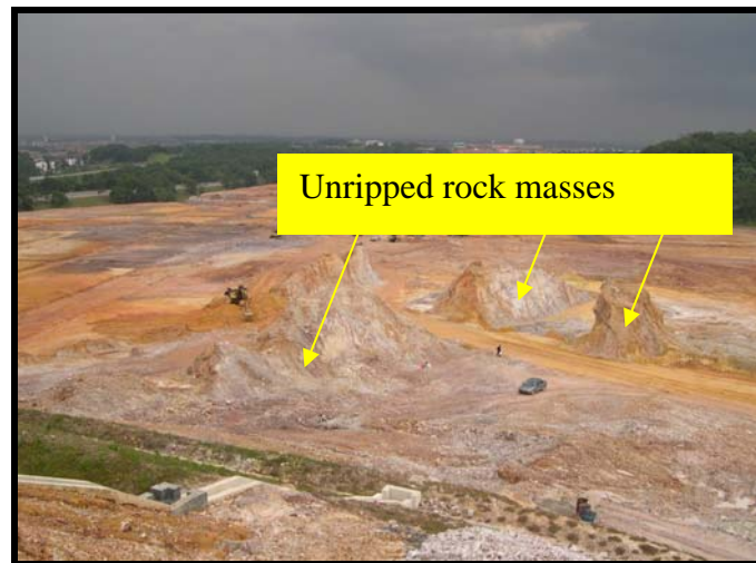
Figure 5.2: Protruding rockmass that could not be ripped by a CAT D9 in Bukit Indah site
