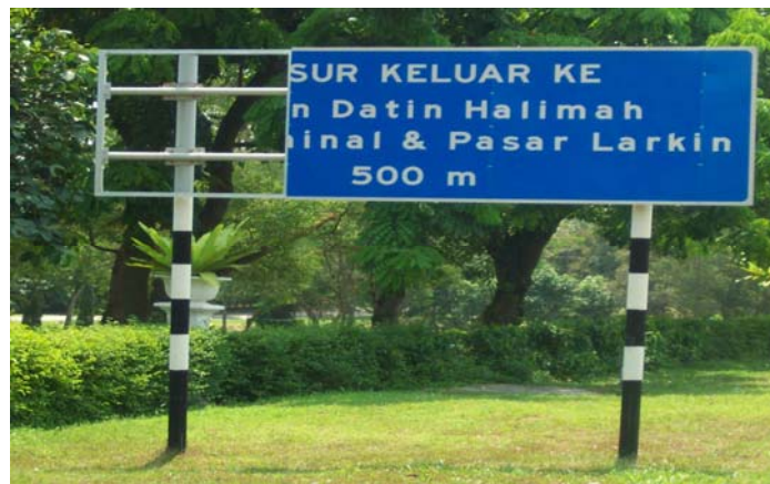
Fig 4: Missing part of the signage
