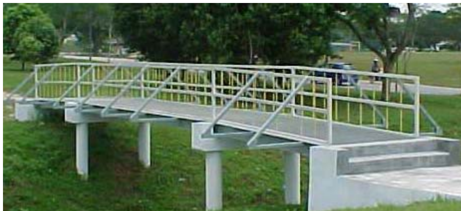
Fig 2: GFRP footbridge at the Universiti Teknologi Malaysia
