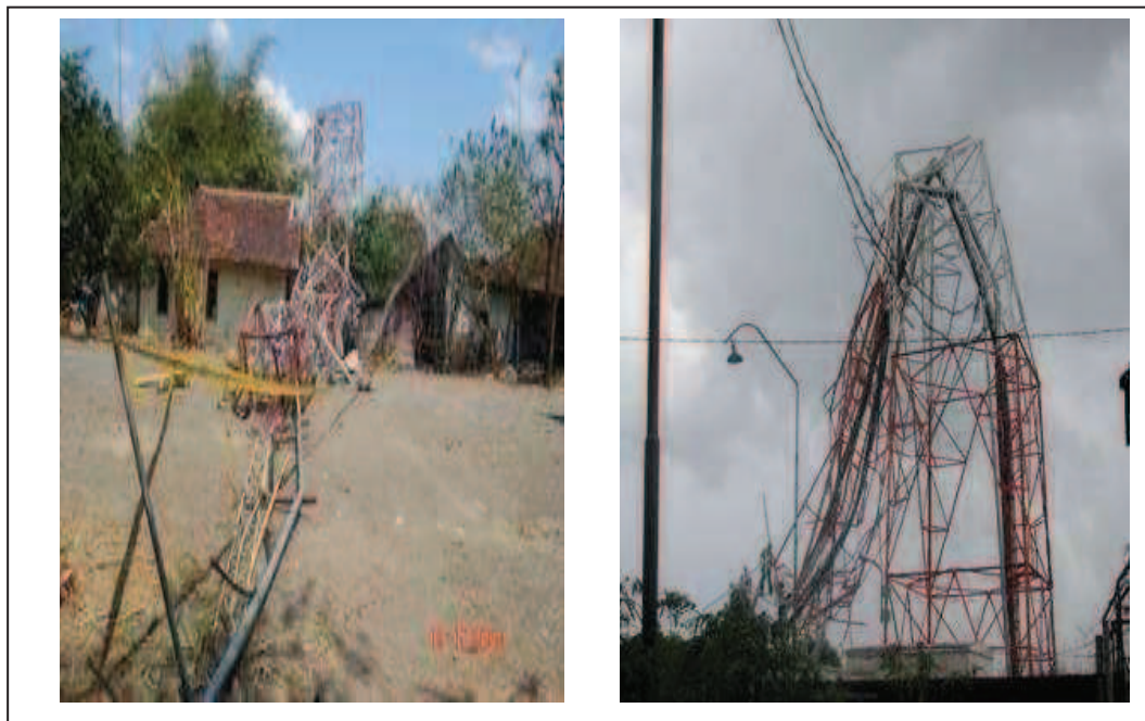
Figure 1.3 Collapsed of tower structure after an earthquake event in Indonesia (PT. XL Axiata Tbk., Indonesia 2011).
