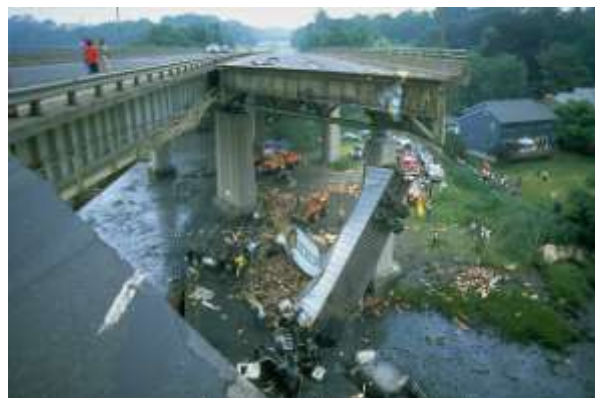
Figure 1.2 Collapse of Mianus River Bridge in Connecticut in year 1983(Morgan, 1983).
