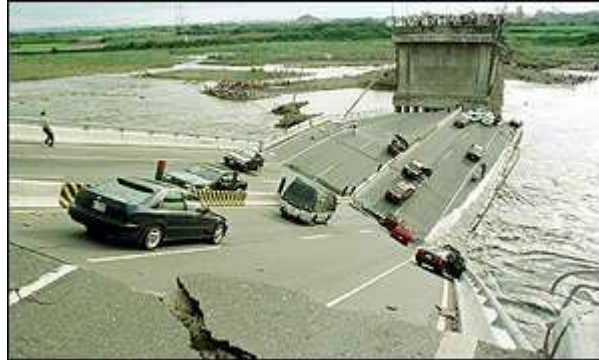
Figure 1.1 Collapse of Kaoshiung-Pingtung Bridge in Taiwan in year 2000(BBC NEWS, 2000).
