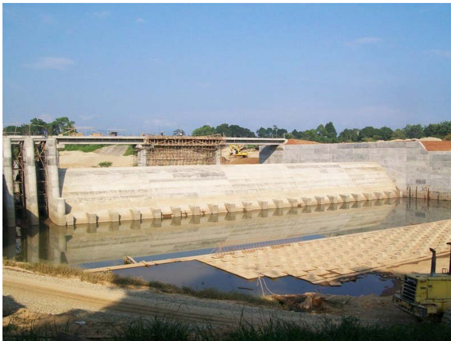
Figure 1.2. Weir Downstream of Air Lakitan Multipurpose Dam
