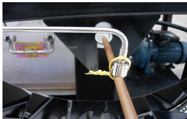
Figure 4.11: Thermocouple attached on Absorber
