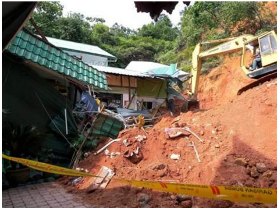
Figure 1.2: Landslide Event at Hidayah Madrasah Al-Taqwa in FELCRA Semungkis
