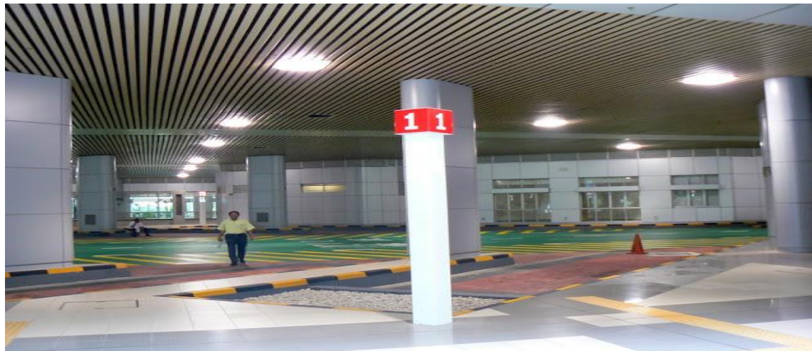
Figure 1.4 : Bus stop without a ramp for disabled people to ride a bus.
