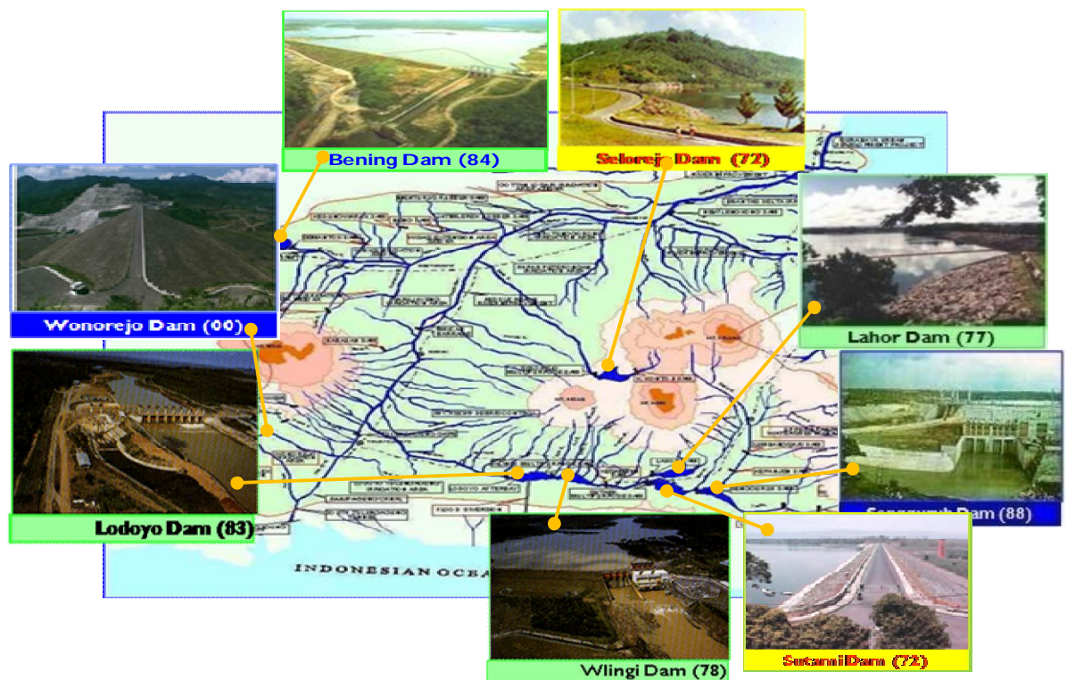
Figure 1.1 Dam Reservoir Infrastructure in Brantas River basin, East Java
