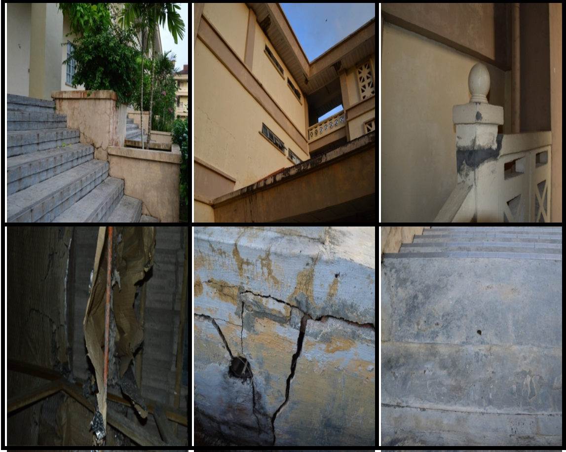
Figure 1.1: M47 Building for Faculty Civil Engineering
