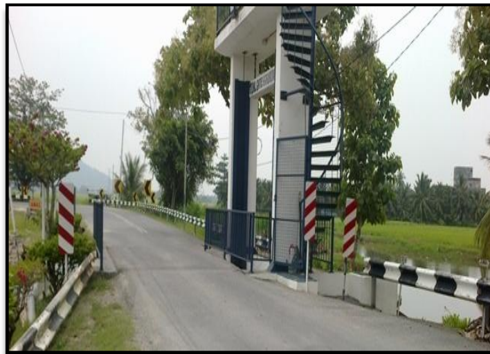
Figure 1.3: The irrigation system for paddy field that narrowing the existing road
