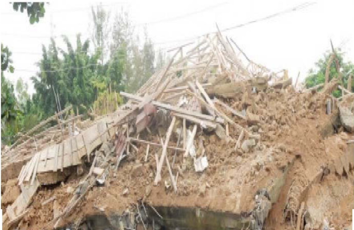
Fig.1.1 Catastrophic collapse at Ikole Street, Abuja of 11th August 2010 (courtesy The Nation on line)
