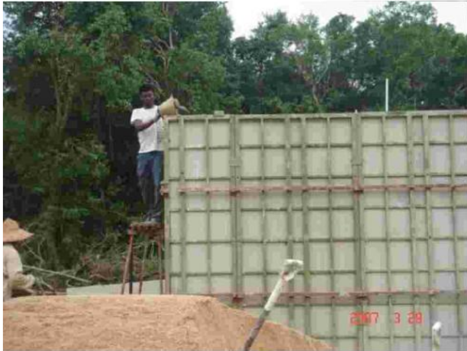
Figure 1.1 Concrete the wall in FTW system
