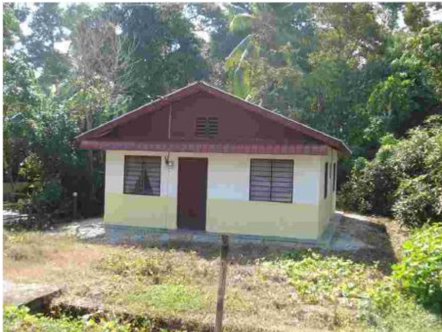
Figure 1.2 Completed single storey house, constructed by FTW system
