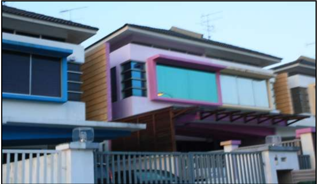
Figure 1.2: Type of double storey house (Licuala Ray)
