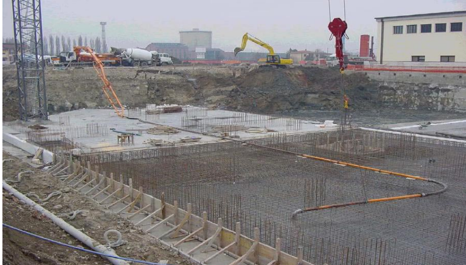
Figure 1.1: The casting of large area of concrete slab [4]
