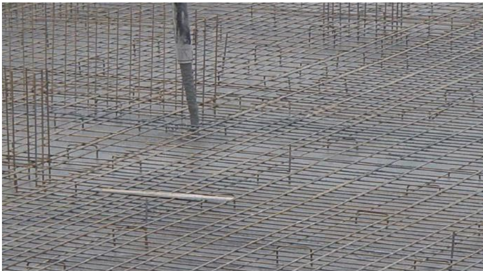
Figure 1.2: Concrete slab with dense reinforcement [4]
