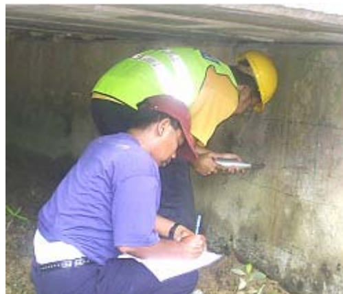
Figure 5: Rebound hammer test conducted on selected abutment
