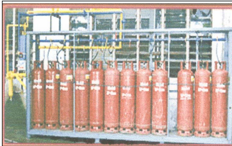
Figure 2.3: Installation based on Manifold System (Min, 1997)
