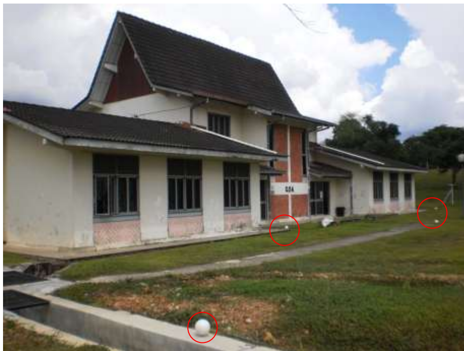
Figure 5: Spheres placement as control point
