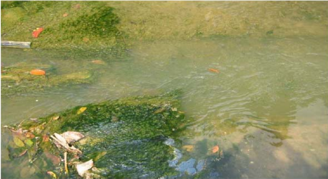
Figure 5.13: Aquatic growth and sedimentation in the channel
