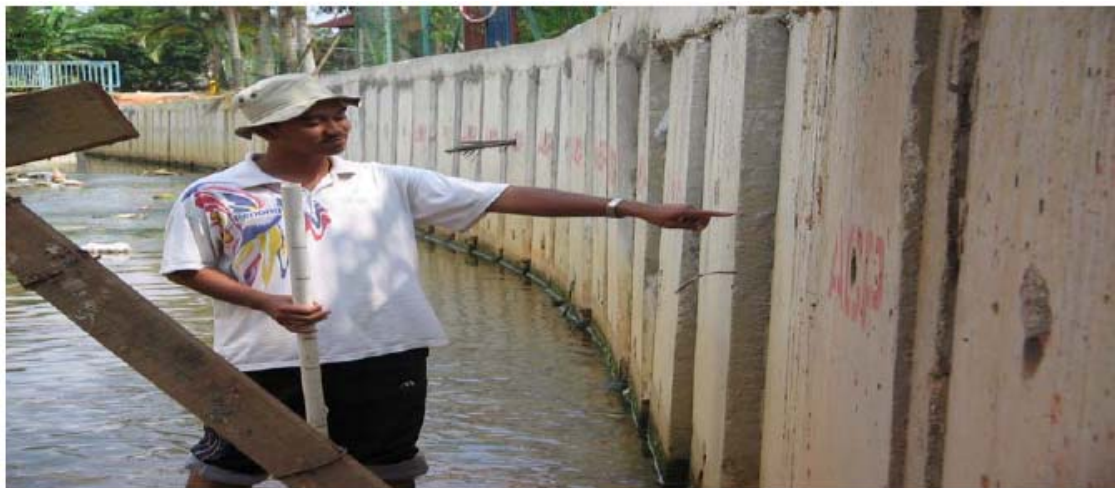
Figure 5.10: Uneven sections during construction which can cause sudden contraction
