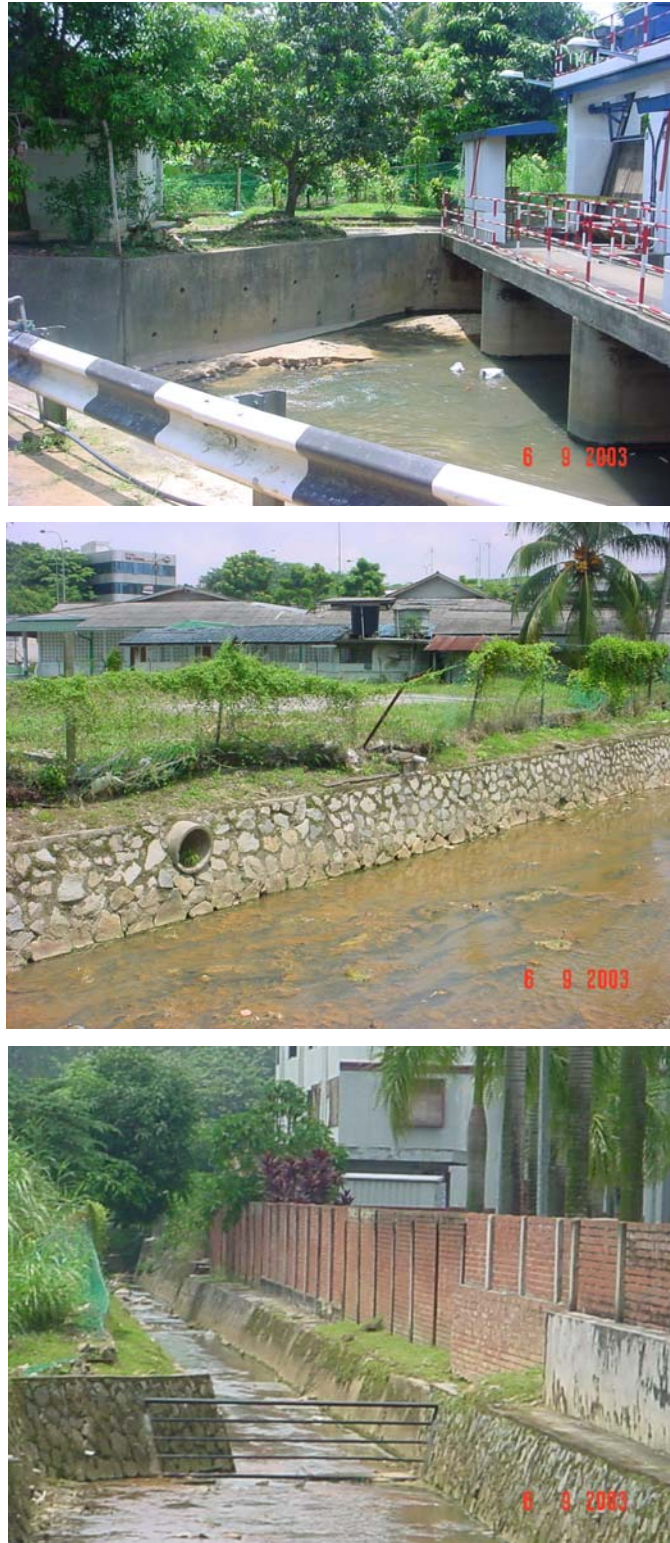
Figure 5.1(b): Pictures of Sg Segget Channel and Affected Areas
