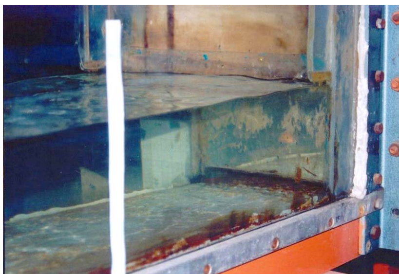
Figure 3.12 Plastic gate at the end of flume
