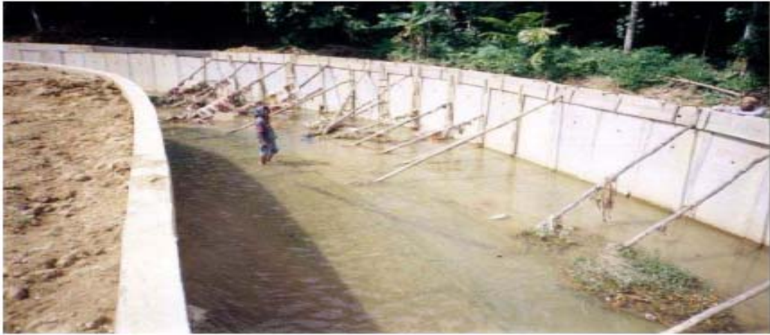
Figure 5.9: The critical sections were replaced with pre-cast concrete channels
