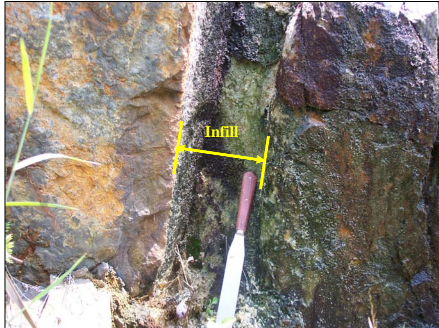
Figure 4.1: Filled joint system with no banding of weathering grade across the infill and joint blocks
