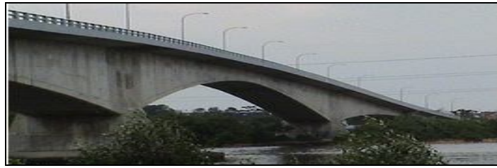
Figure 1.6 Permas Jaya Bridge, Johor
