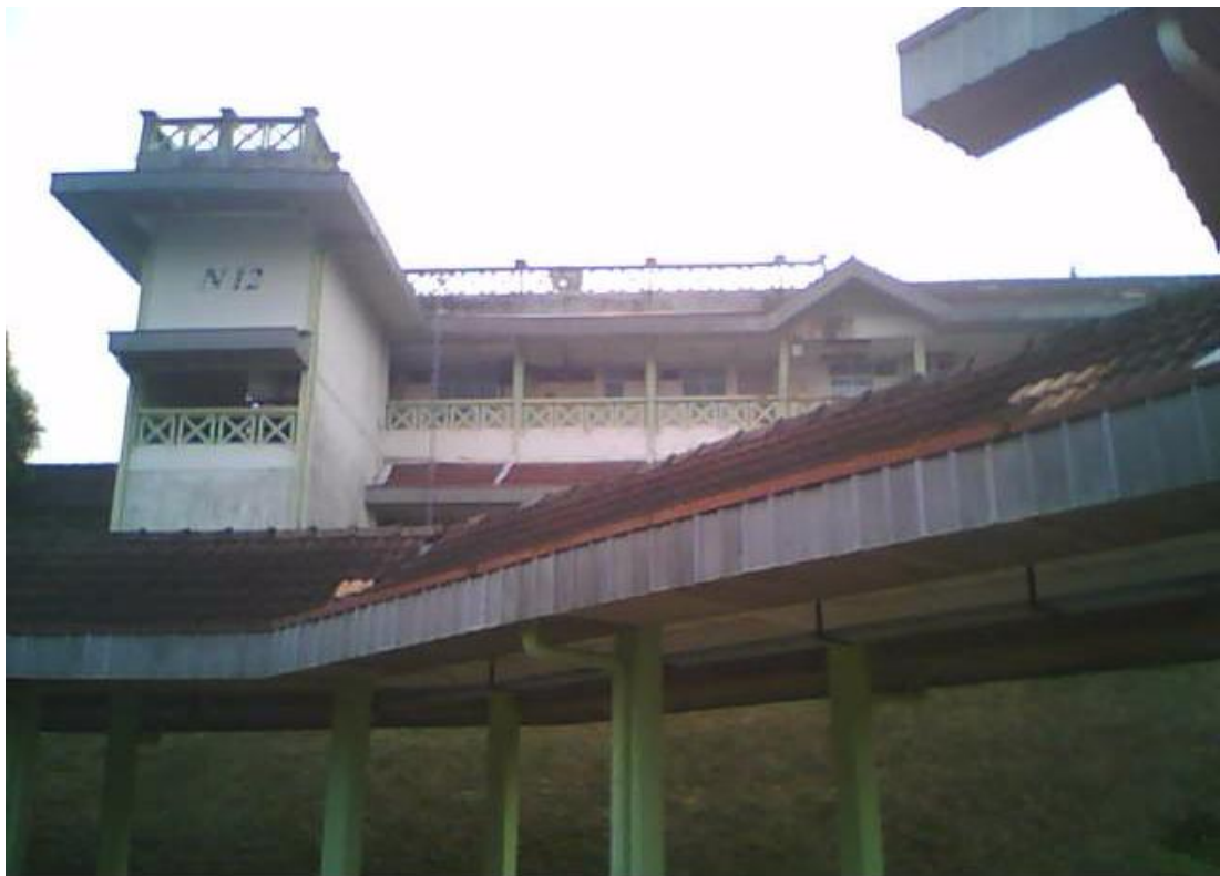
Figure 3.1: N12 Building. Parabolic concentrator is located at top of the building.
