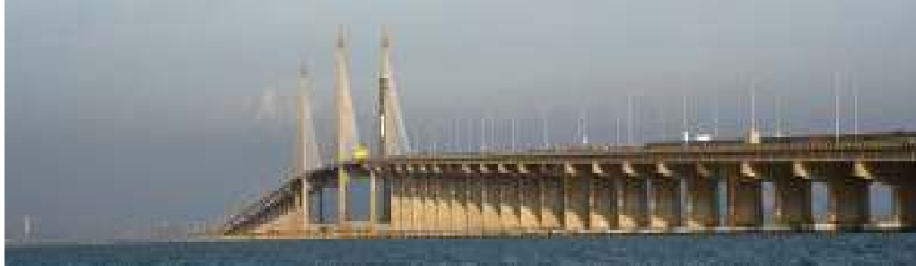
Figure 1.1: The Penang Bridge ( www.en.wikipedia.org ).
