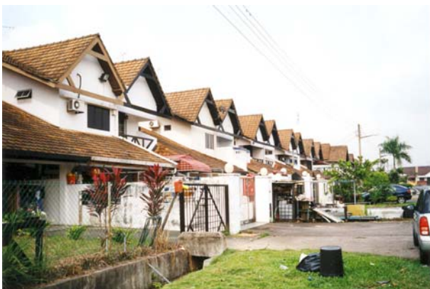
Fig.1. Terraced houses in case study area
