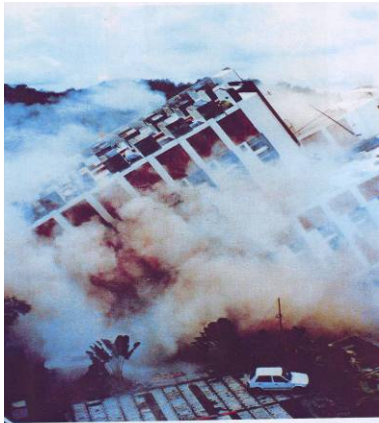
P3 Photograph showing Block 1 toppling over with The Block Tower translating approximately 3 to 4 floors relative to Front Tower
