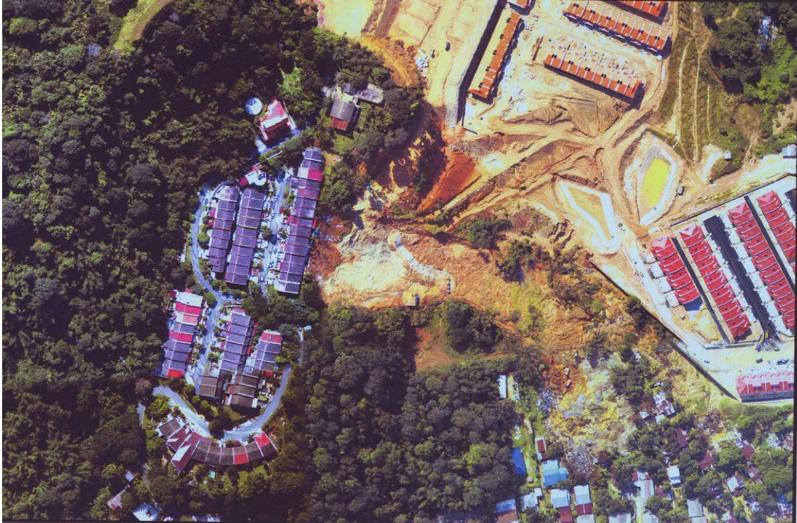
Figure 5.9 : Zoo view – kampong pasir landslides looking from aerial view
