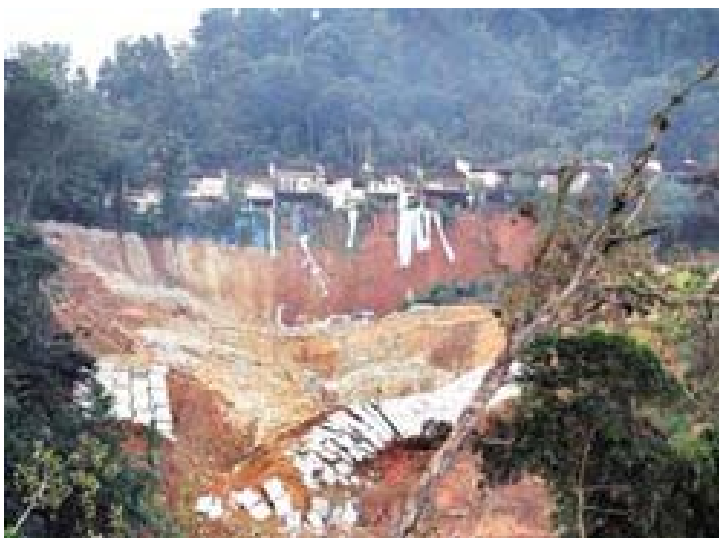
Figure 5.8: Retaining wall failed in zoo view development, it flow to kampong pasir area and ruined 3 blocks of long house
