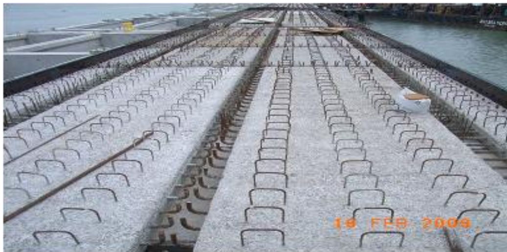
Figure 1.3: Shear Key in Precast Member
