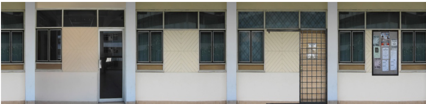
Figure 3: Part of the joint rectified photos
