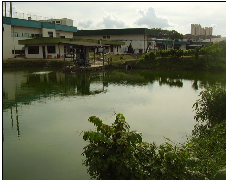
Figure 1.4 : Facultative pond located beside the concrete batching plant
