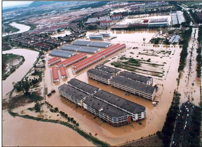
Figure 1.3: Flooded area at Shah Alam, Selangor due to high tide.
