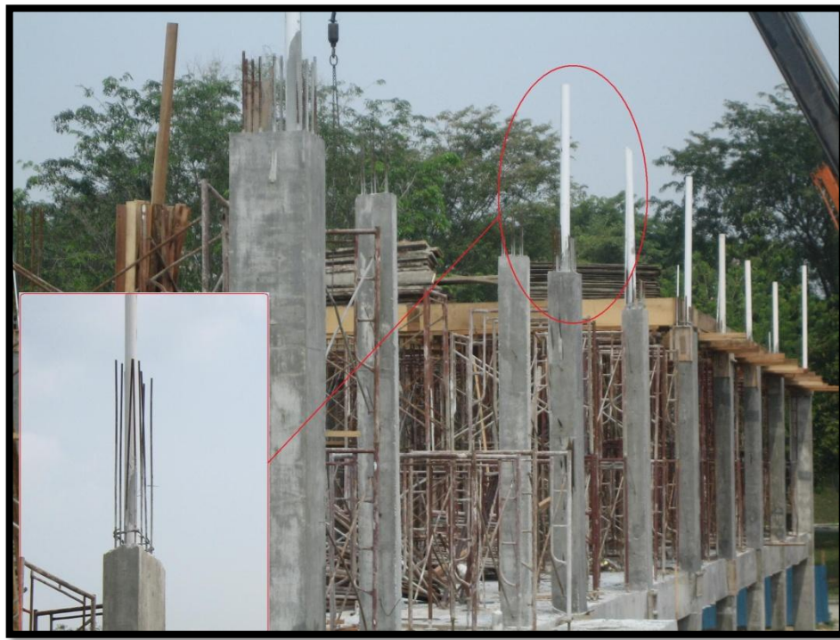
Figure 1.1: Rain Water Pipe Is Positioned Inside Columns
